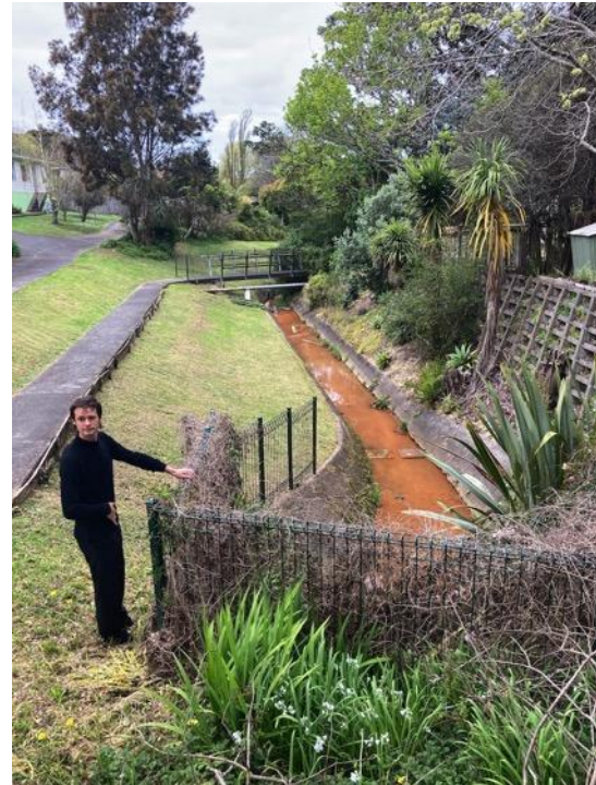
Figure 25: Walkway and bridge from Celina Place
